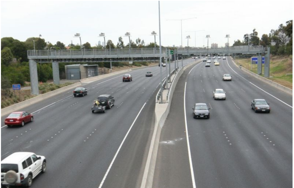
Figure 8 - Toll gantries on the Tullamarine Freeway section of Melbourne's CityLink – by Marcus Wong
