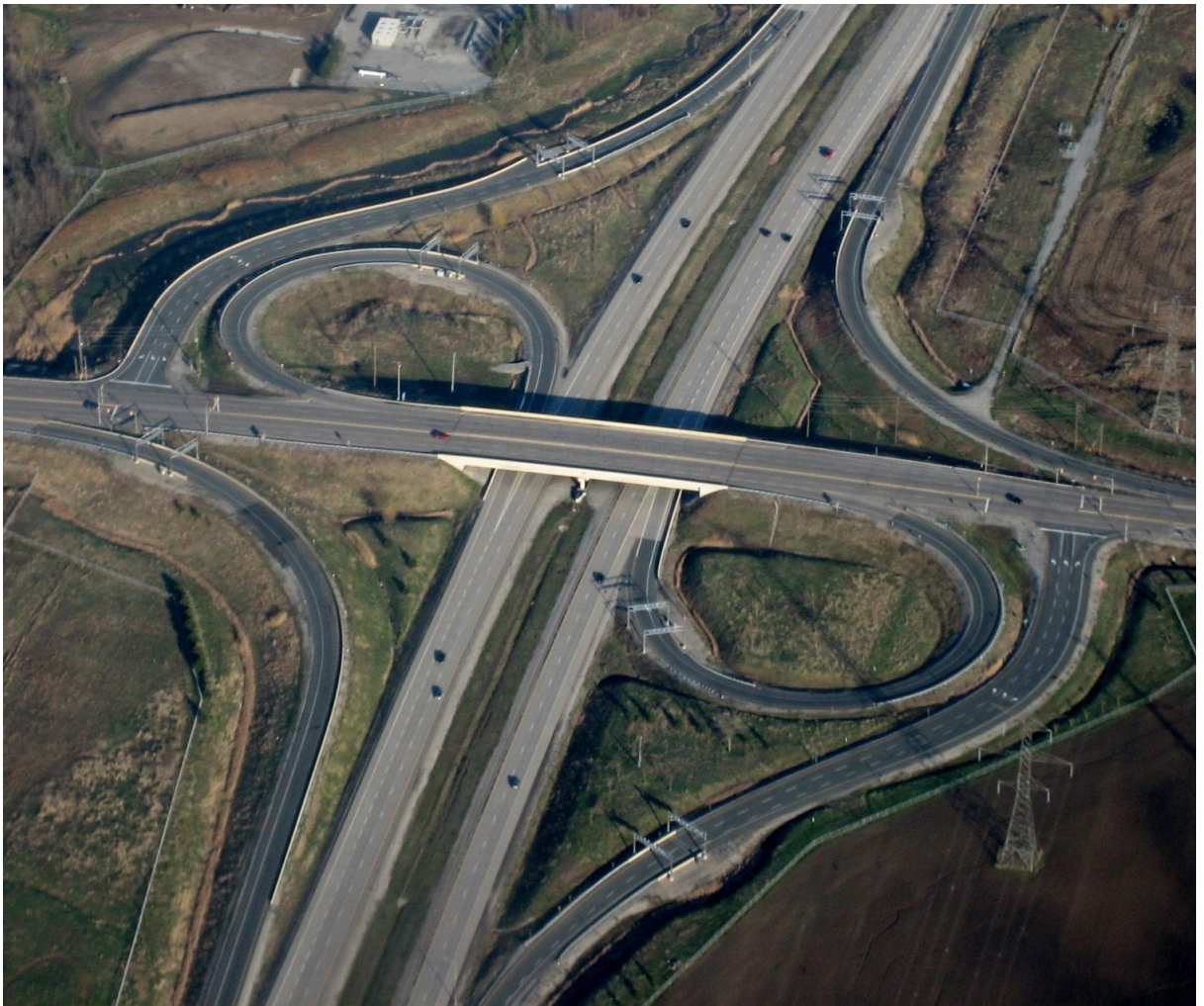
Figure 9 - Highway 407 and Derry Road, facing southwest - By SimonP
